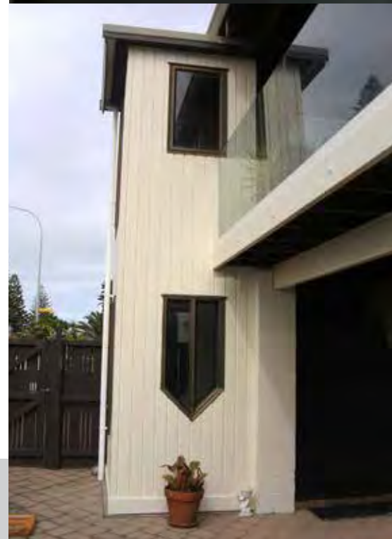
External Lift Shaft
