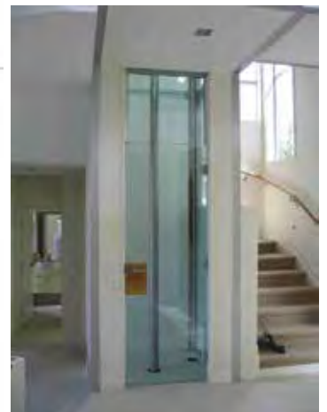
Glass door showing stainless steel ram
